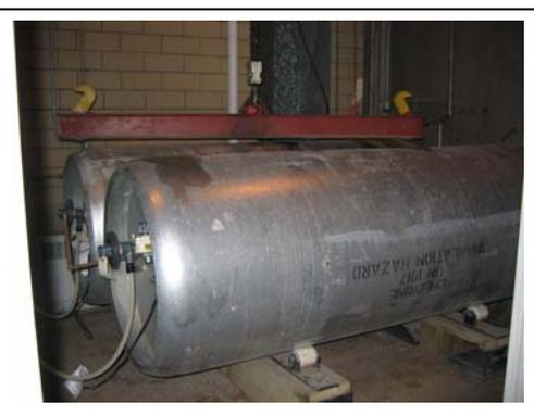
**In-use chlorine tanks stored next to operator room, main bldg.**
