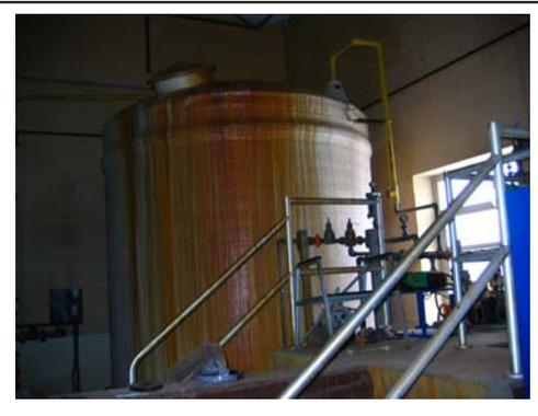
**6000-gallon container of ferric chloride located in CSPT 2 bldg.**
