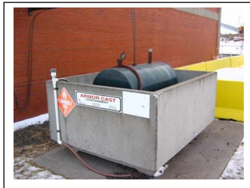
**290-gallon drum of diesel fuel stored outside within a cement containment area.**
